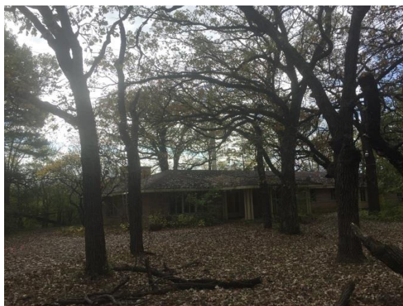
The Kilburn Building on the Elgin-owned former Fox River Country Day School Campus is one of three dormitories set for demolition. (Mike Danahey/Courier-News )
